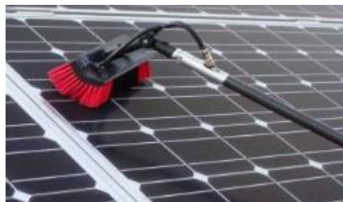
Figure 3-19 Manual Dry Cleaning
