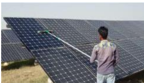
Figure 3-18 Manual Dry Cleaning
