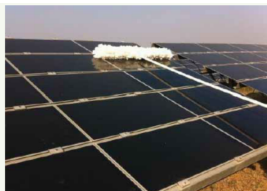
Figure 5-3 Module cleaning Using Dust Broom
