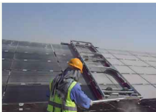
Figure 5-2 Module cleaning Using Brush Trolley 1
