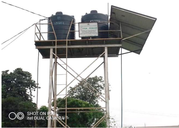
Plate 5.7: A borehole provided for Siun located in front of the Olu of Siun land palace
