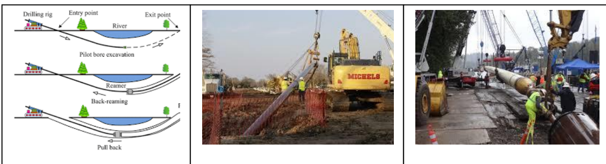
Figure 2.5: Horizontal Directional Drilling process
