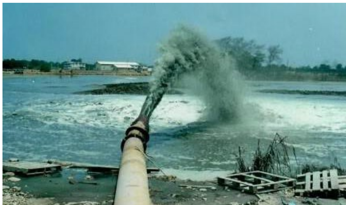
Dumping of sediments dredged from the piers in the sediment ponds, between 2004 and 2009.
