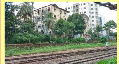
N1-Northern Residential Building
