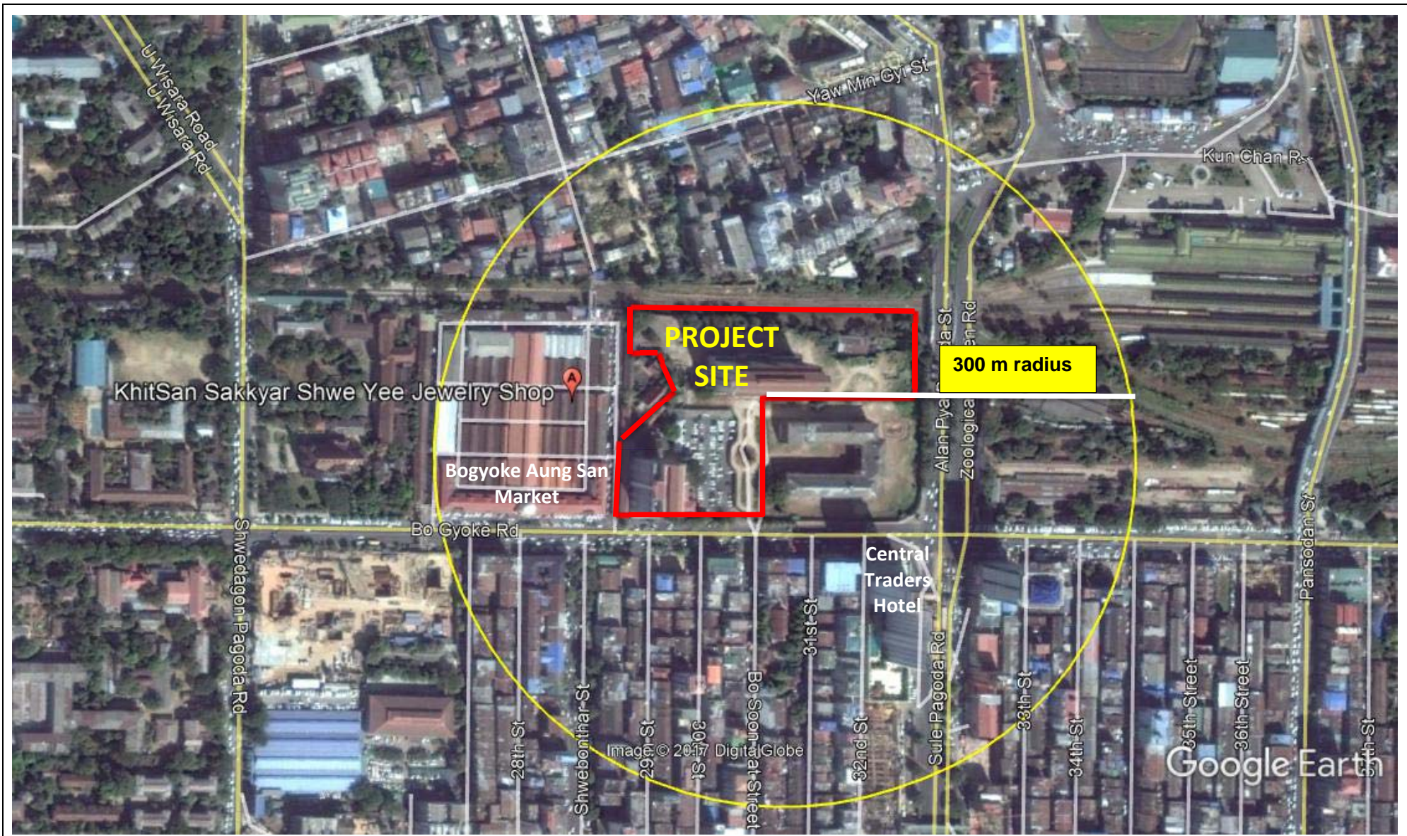
Figure 4.3: Aerial View of Site and the Surrounding Areas within a 300 m Radius
