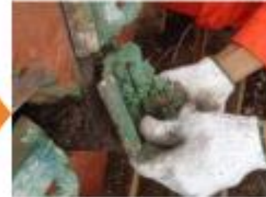
Unscrew bolts & remove fascia edge (6,8)
