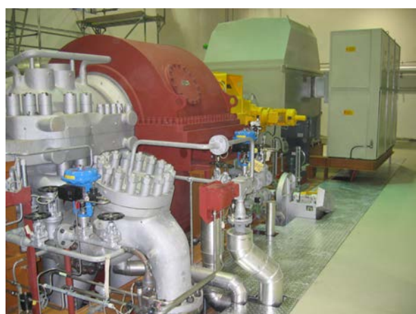
Picture 7: Steam turbine turbo set
