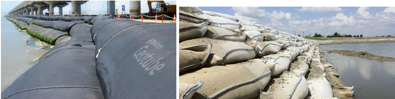
FIGURE 1 – TYPICAL SHORE PROTECTION WITH GEOTUBES AND BAGS
