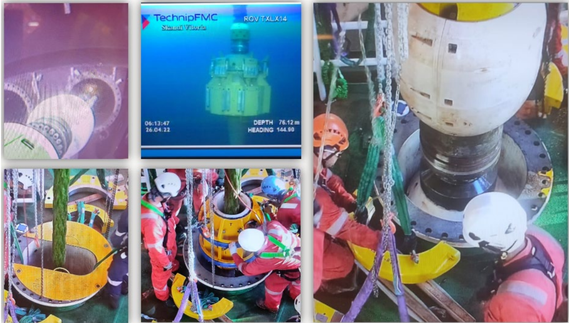
Figure 4.14: SURF installation – flexible lines connection with the Coral South FLNG
