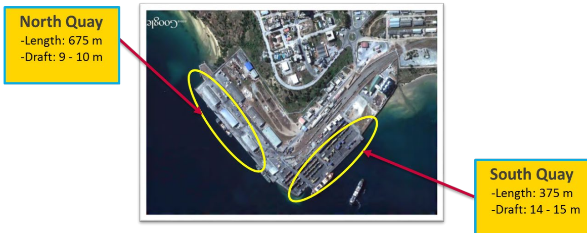
Figure 4.6: North and south quay in the Port of Nacala
