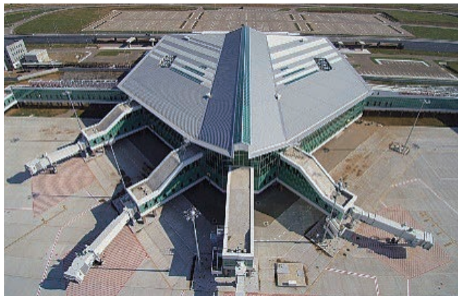
写真提供: New Ulaanbaatar International Airport LLC
