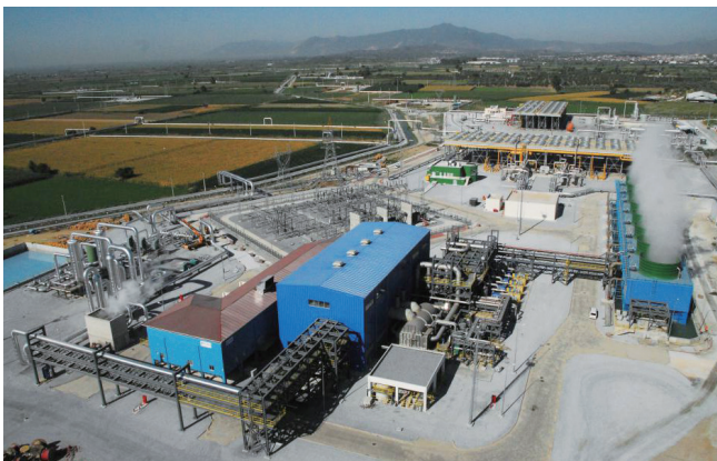
Photograph courtesy of Gurmat Elektrik Uretim A.S.
