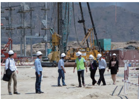
Scene from On-site Visit to a Construction Site
