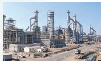
Photograph courtesy of Reliance Industries Limited
