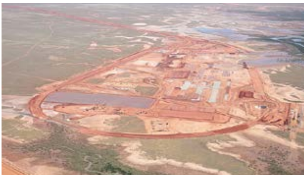
Photograph courtesy of Roy Hill Holdings Pty Ltd
