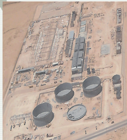
Photograph courtesy : Amman Asia Electric Power Co.
